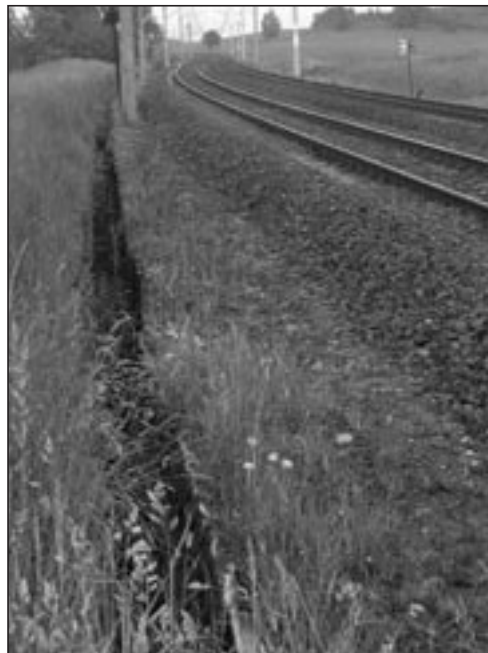
Fig. 4. So-called Krakow-type open channels, serving to drain the railway line embankment, are a barrier for amphibians and other animals
