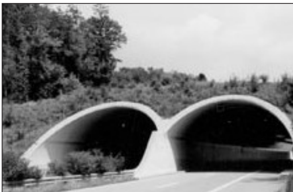
Fig 9. Belgium. A bridge over the highway between Brussels and Luxemburg in a forested region. It is only 8 meters wide, but very well managed. The bridge surface is leveled with the surrounding forest. Roe deer use this bridge
