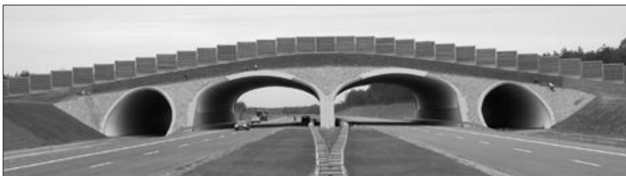
Fig. 4. The view of the completed ecological bridge
