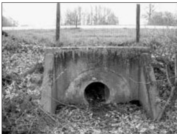
Stubwall under viaduct
