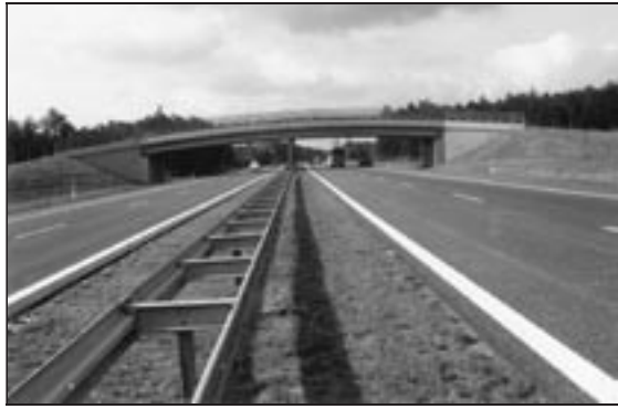
Fig. 2. A bridge with an open-work fence at km 217.7, situated amidst forests. ‘Funnels’ are not planted with trees or bushes
