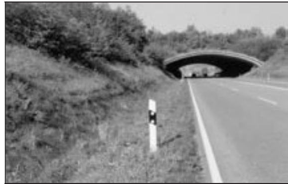
Fig 10. Germany. Road B31. One of several wildlife bridges, 33 meters wide. The road surface near the bridge was lowered
