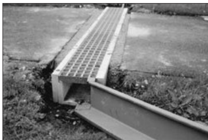
Fig. 8. Culvert on one of the roads in Belgium, built even with the road surface
