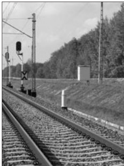
Fig. 1. Depicts a UOZ-1 device installed by the track-way and the linear self-blocking container next to it
