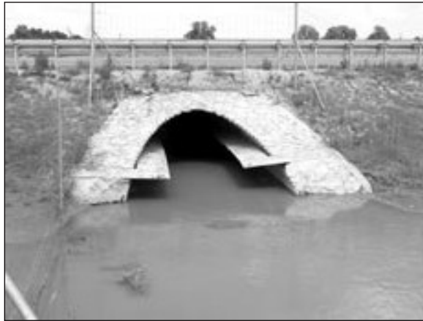
Fig. 7. An example a pass for amphibians and small mammals under highway A2
